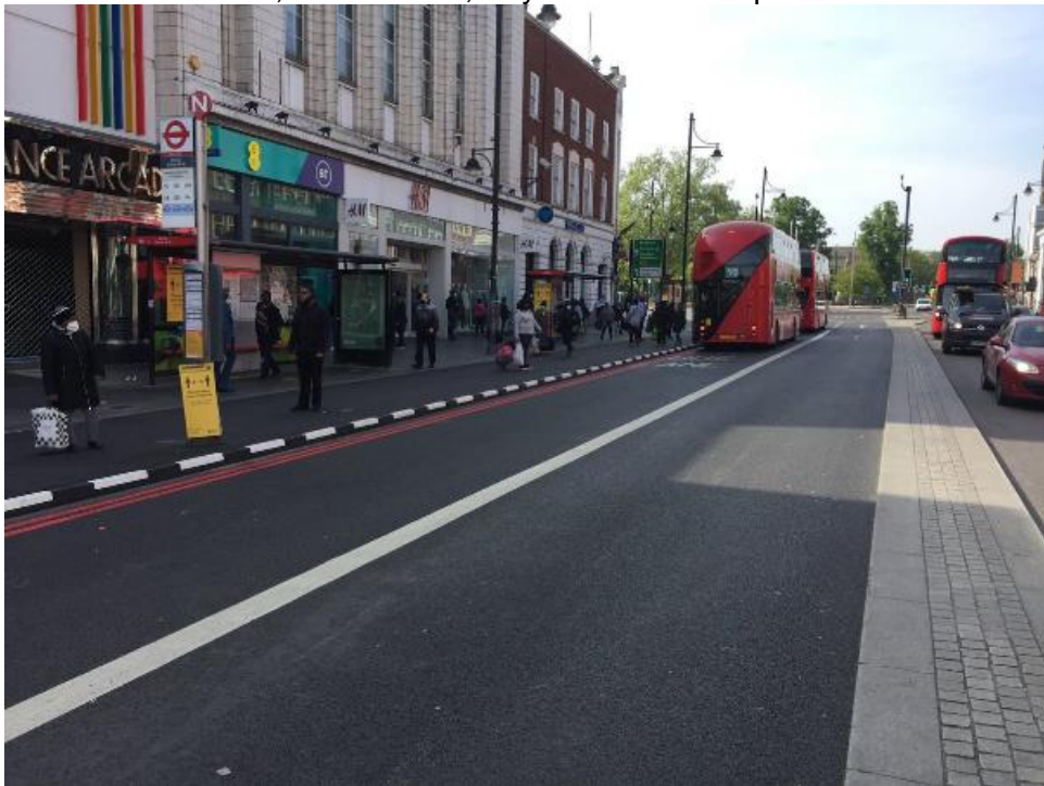
Example of Temporary Cycle Build out at a bus stop in Paris
